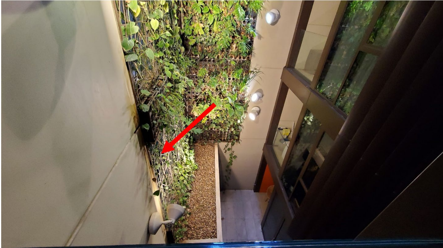
view of atrium from level three resident balcony with terrace behind green wall to the left
