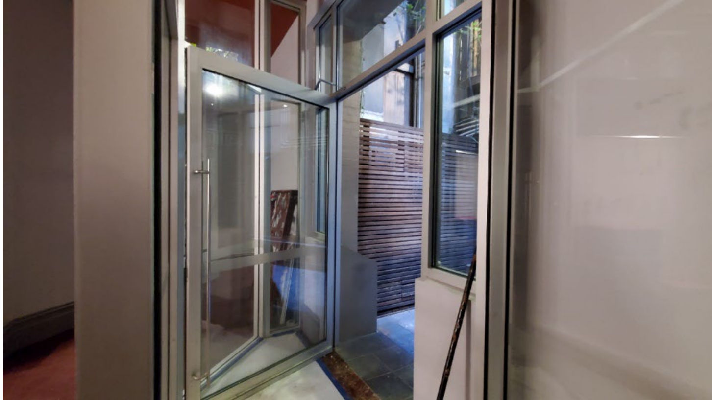
Entry to first floor outdoor terrace
